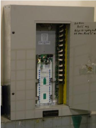
Loeb Electric installed a low voltage panel to eliminate wasted energy in the PSB facility. The panel supplies lighting in spaces based on occupancy and day lighting conditions.
